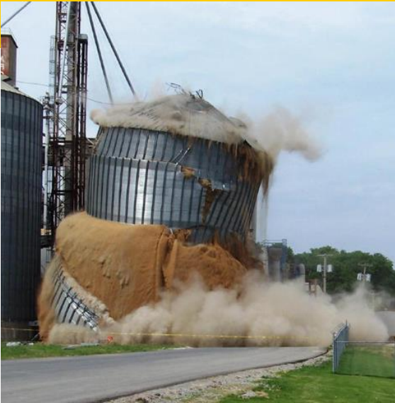
Bridging transfers load to the bin wall
